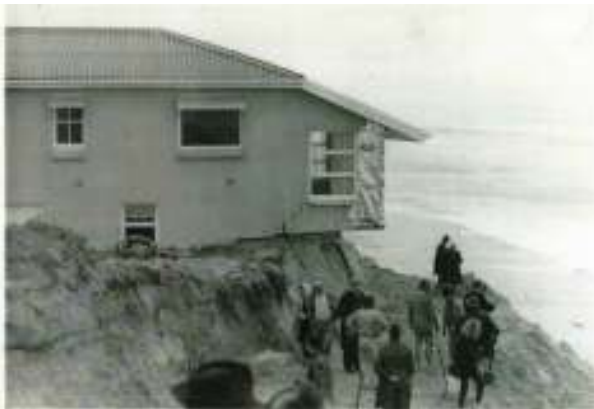
Figure 1; Typical 1960s Gold Coast beach house
