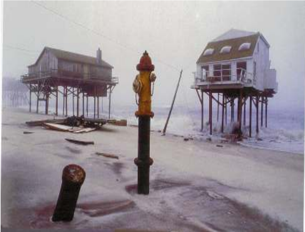
Figure 3 Houses on beach after storm erosion and rapidly rising sea level on the east coast, USA
